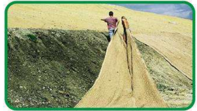
Slope Erosion Control
